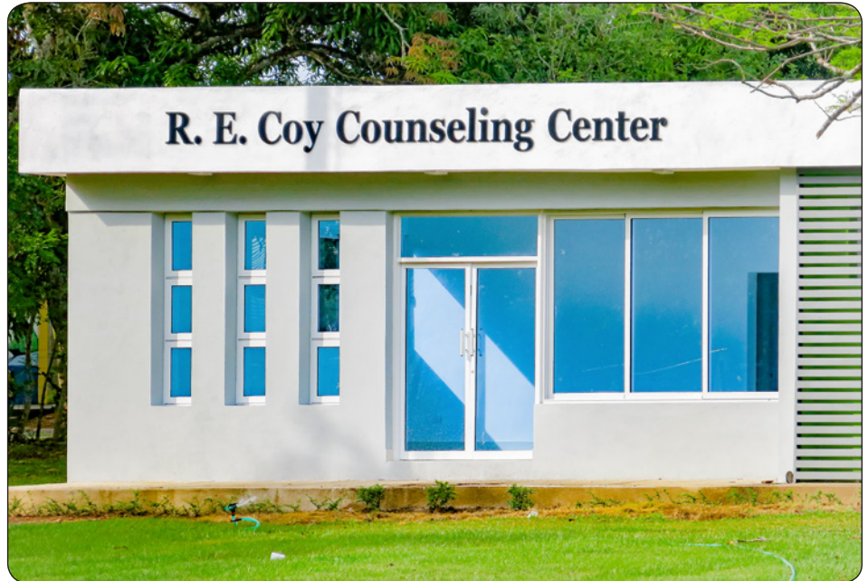
The main entrance to the counseling center section of the new R.E. ‘Robert’ Coy Counseling Center & Elder G.W. Brown Medical Clinic. The clinic building is located on the campus of the Las Palmas Children’s Village in the Dominican Republic. The clinics were opened and dedicated during a ceremony held in May of 2019.
