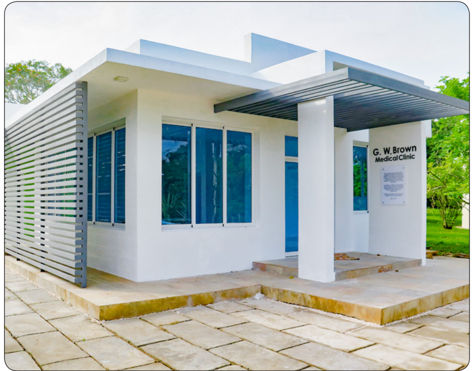
The main entrance to the medical clinic section of the new R.E. 'Robert' Coy Counseling Center & Elder G.W. Brown Medical Clinic. The clinic building is located on the campus of the Las Palmas Children's Village in the Dominican Republic. The clinics were opened and dedicated during a ceremony held in May of 2019.
